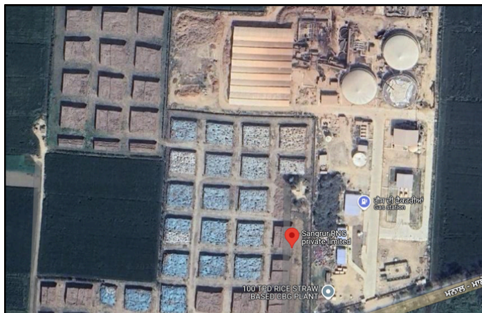
Image of Thermax Bio-gas plant
